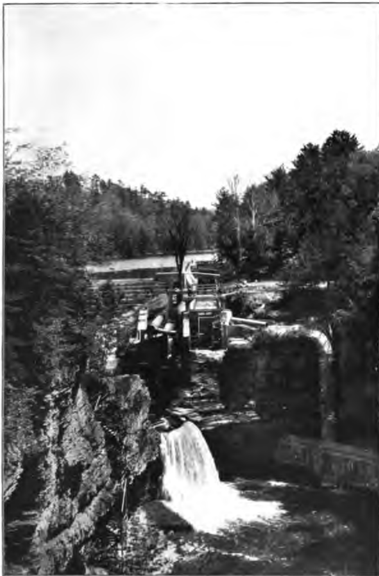
CORNELL HYDRAULIC LABORATORY, ARRANGED FOR WEIR EXPERIMENTS.
