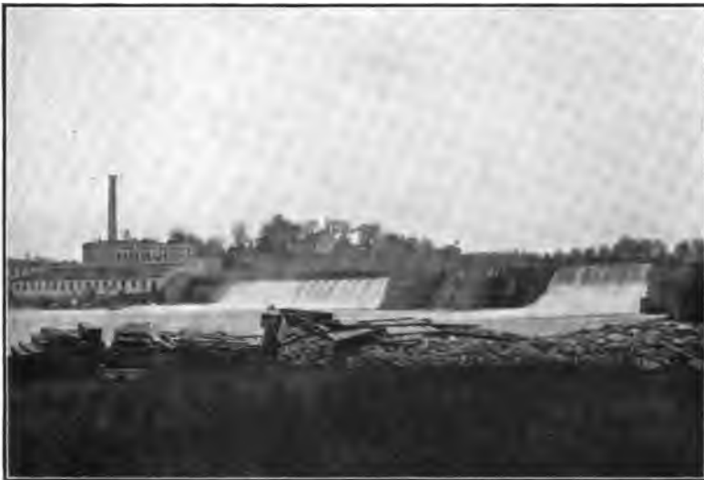
B. COMBINED LOCKS DAM ON LOWER FOX RIVER AT LITTLECHUTE.
