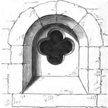
CLERESTORY WINDOW, NOW WITHIN THE BUILDING.
