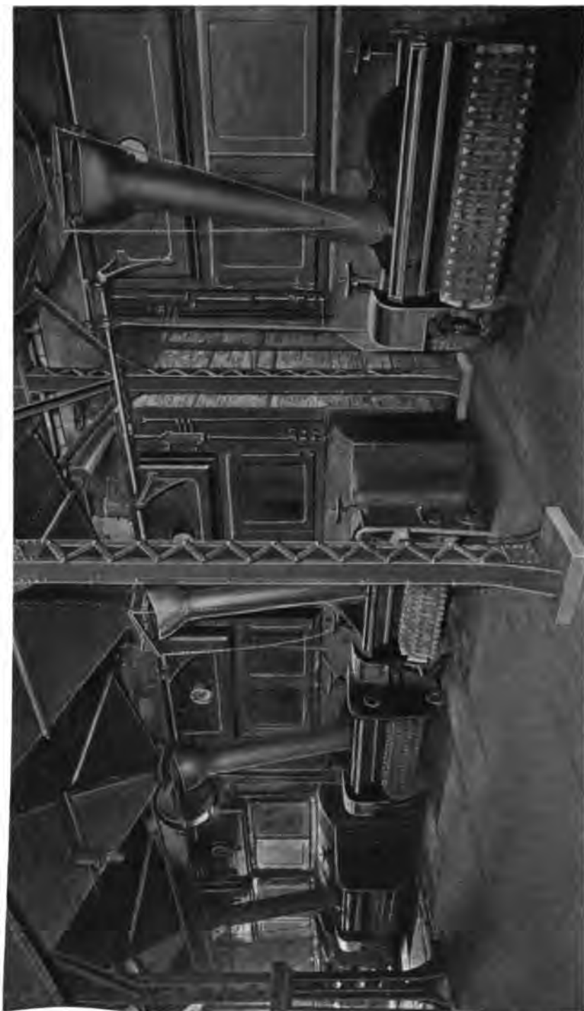
1500 H. P. of Heine Standard Boilers equipped with Laclede-Christy Chain Grate Stokers installed in the Duncan and Newstead Avenues plant of the Polar Wave Ice and Fuel Co., St. Louis, Mo. This company has installed 4250 H. P. of Heine Standard Boilers.
