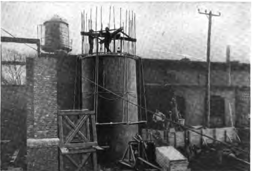
Fig. 111. Completed Base Section of a Concrete Stack.
