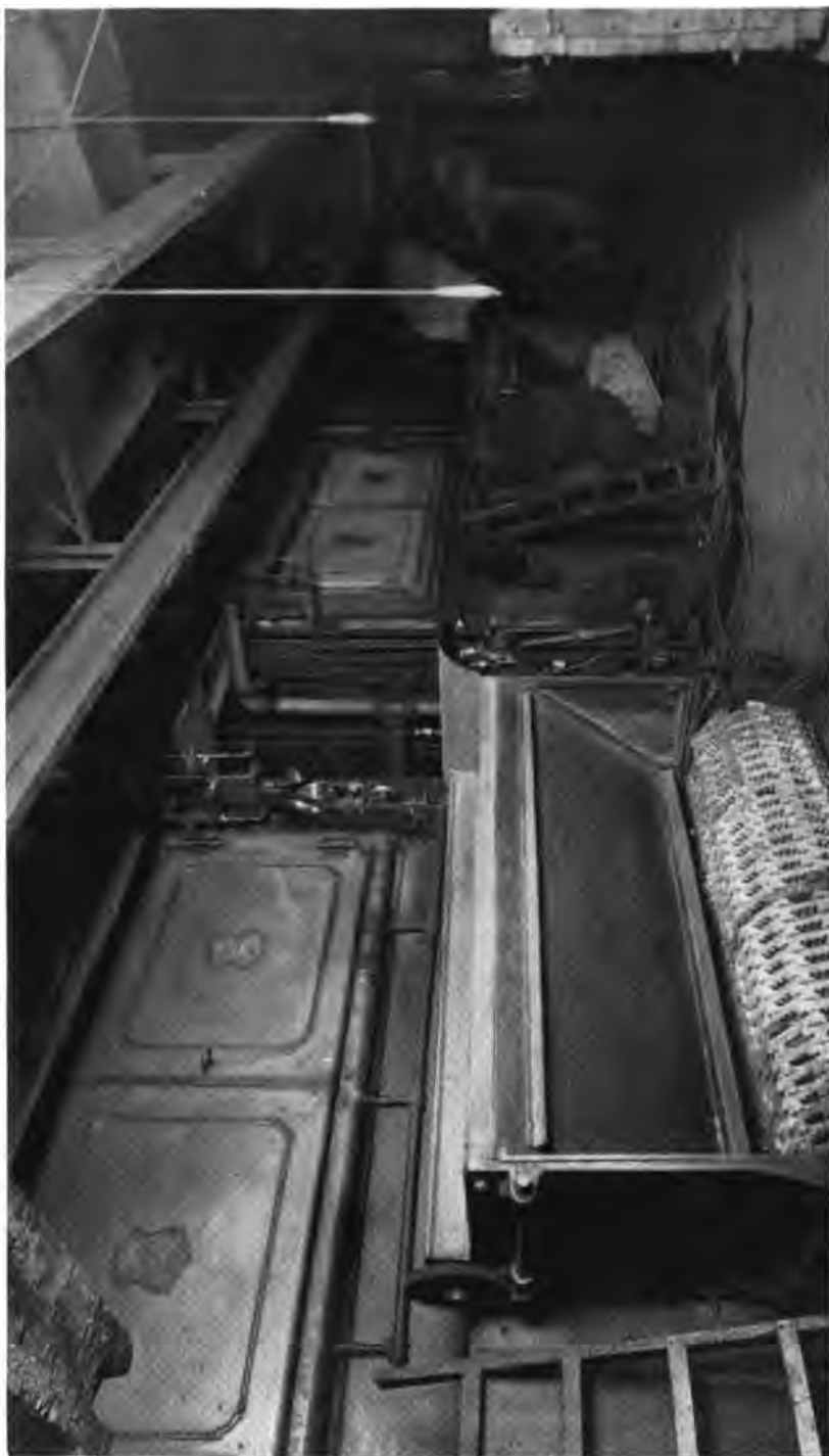
840 H. P. of Heine Standard Boilers equipped with McKenzie Chain Grate Stokers installed in the McCormick Building, Chicago, Ill.
