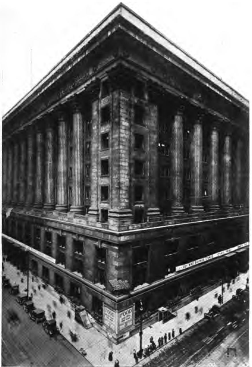
Cook County Court House, Chicago, Ill., containing 1830 H. P. of Heine Standard Boilers.
