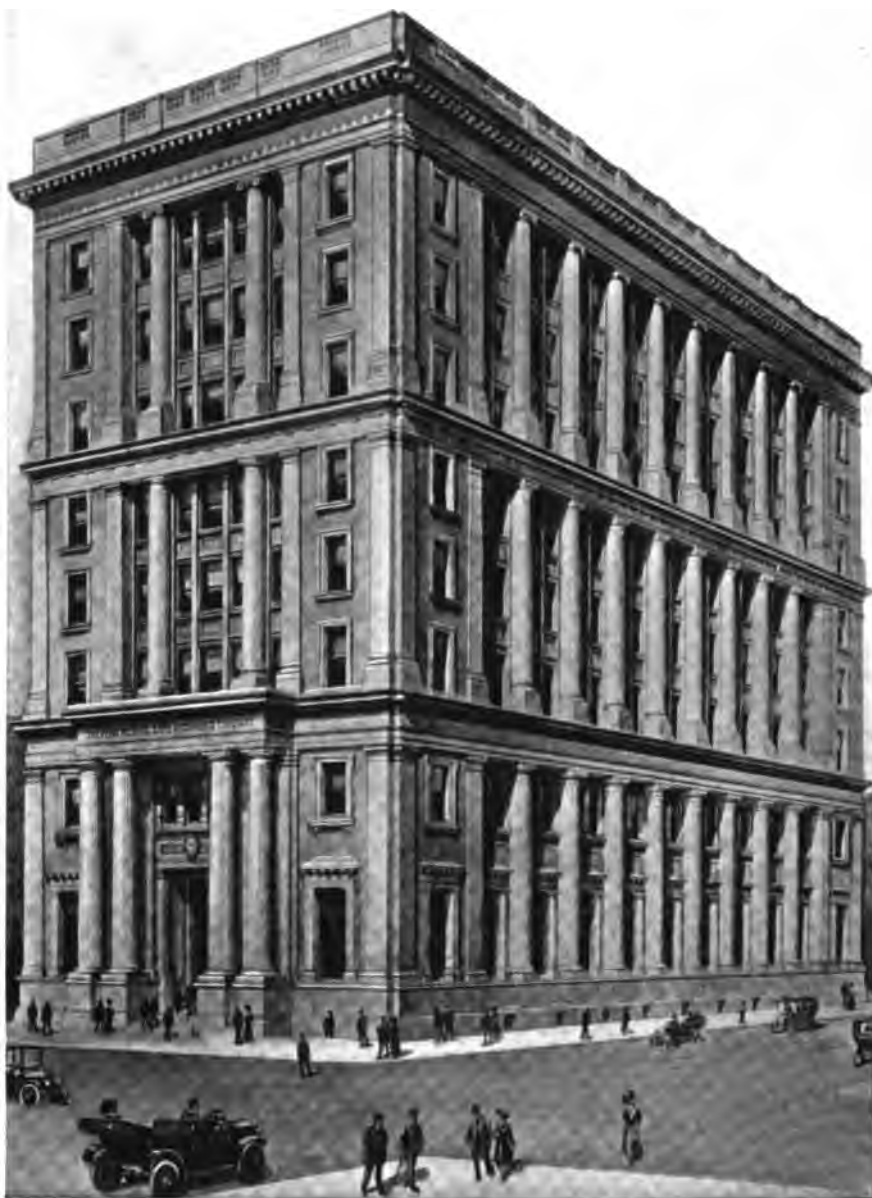
Penn Mutual Life Insurance Building, Philadelphia, Pa., equipped with Heine Standard Boilers.
