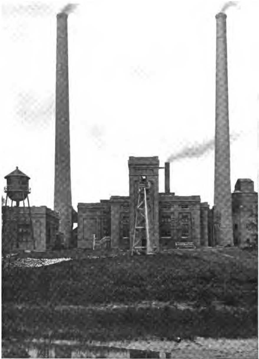
St. Joseph Lead Co., Rivermines, Mo., operating 7000 H. P. of Heine Standard Boilers.
