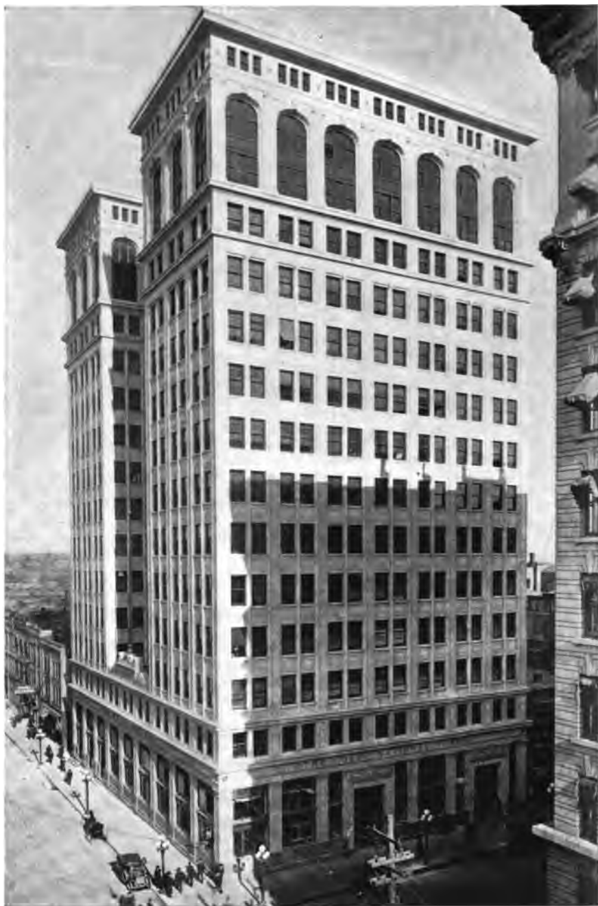
Old National Bank Building, Spokane, Wash., equipped with Heine Standard Boilers.
