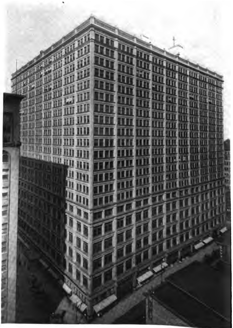
Railway Exchange Building, St. Louis, Mo., operating 1052 H. P. of Heine Standard Boilers.
