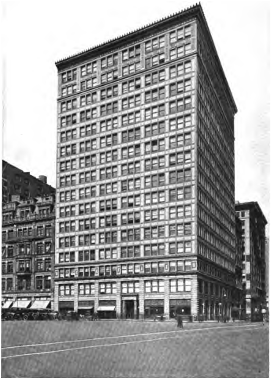
Everett Building, New York City, equipped with Heine Boilers.
