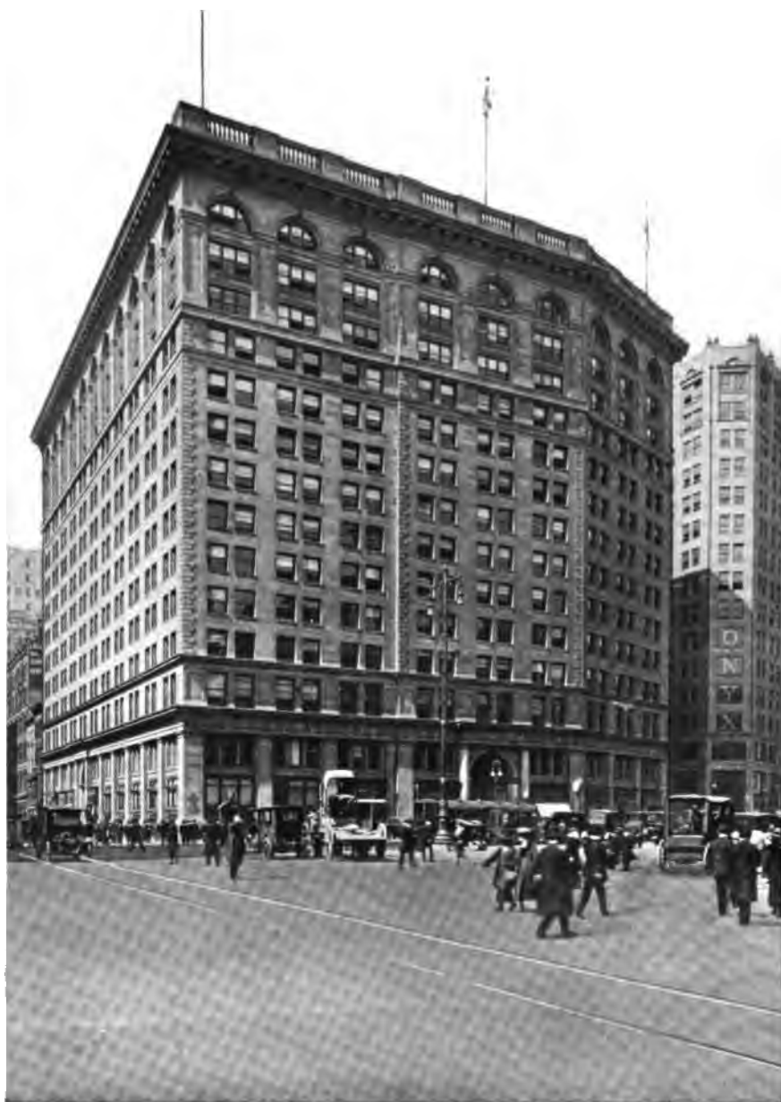
Fifth Avenue Building, New York City, operating 1400 H. P. of Heine Standard Boilers.
