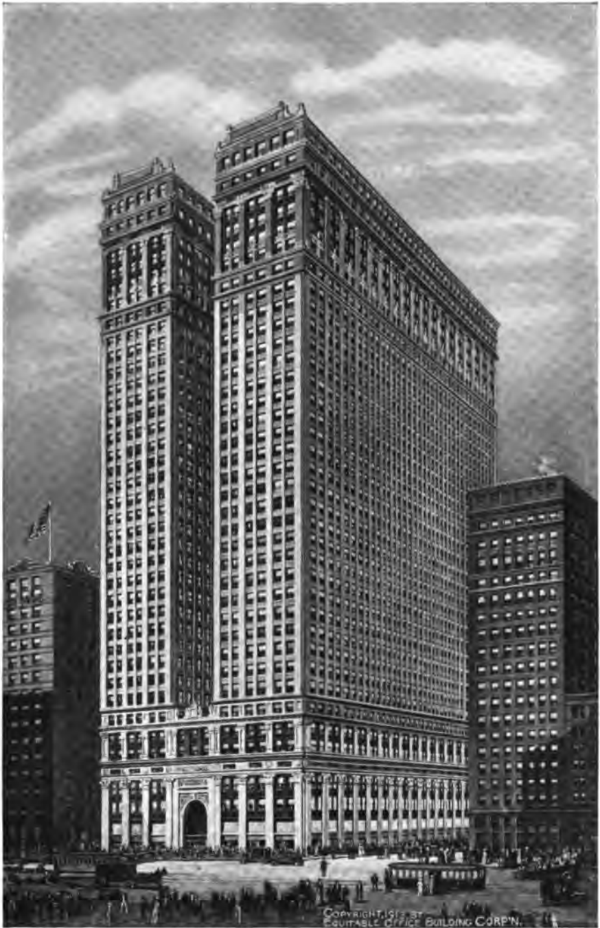
Equitable Building, New York City. 3500 H. P. of Heine Standard Boilers. Tallest Chimney in the World.
