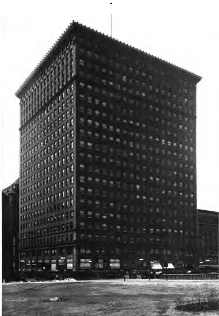
McCormick Building, Chicago, Ill., equipped with Heine Standard Boilers.
