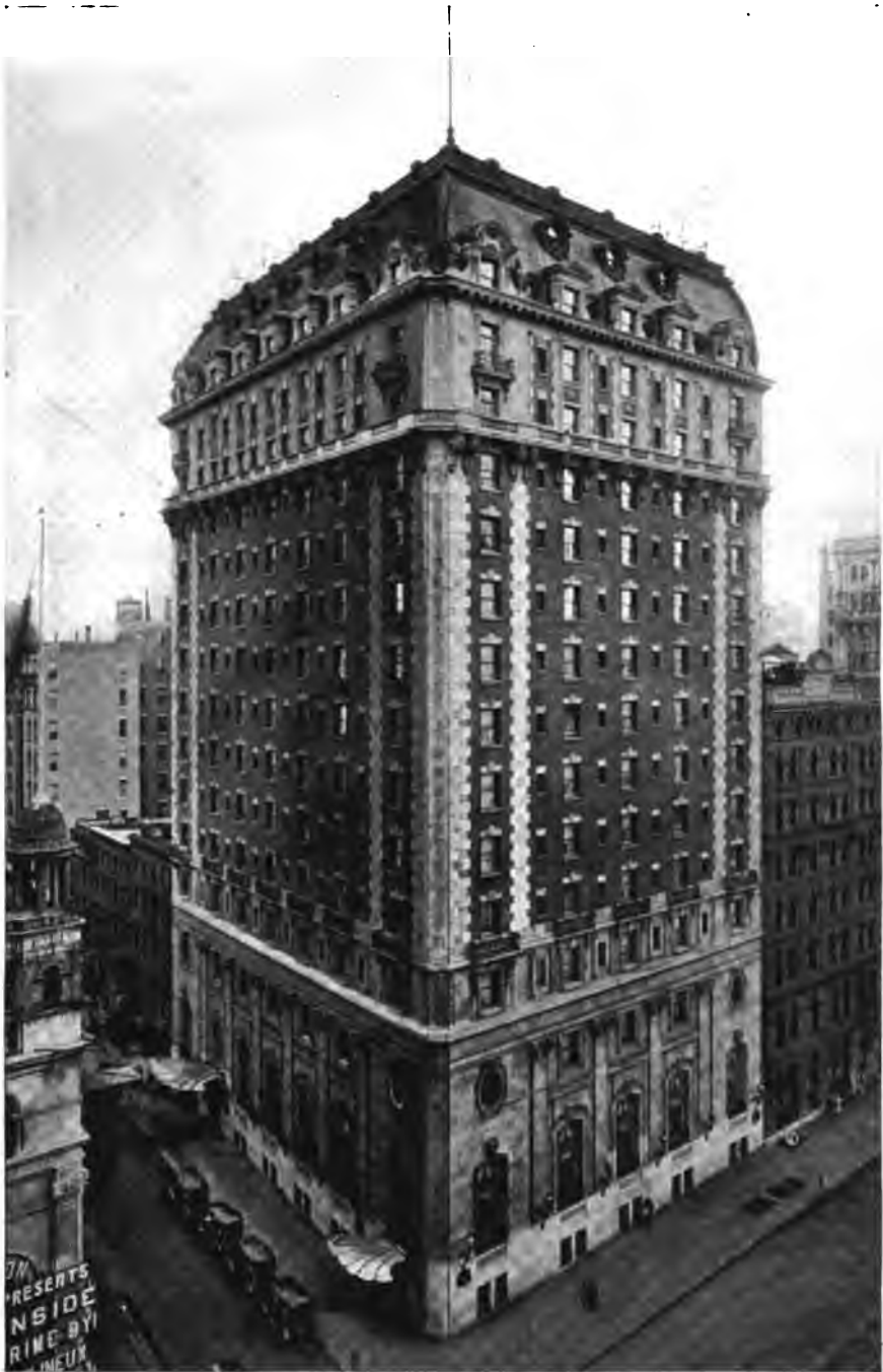
Hotel Claridge, New York City, equipped with Heine Boilers.
