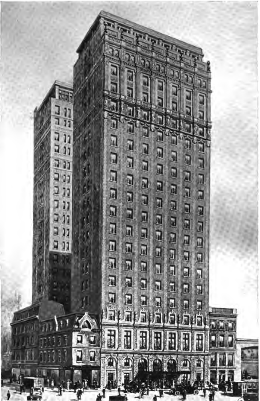
Adelpia Hotel, Philadelphia, Pa., containing four 255 H. P. Heine Standard Boilers.
