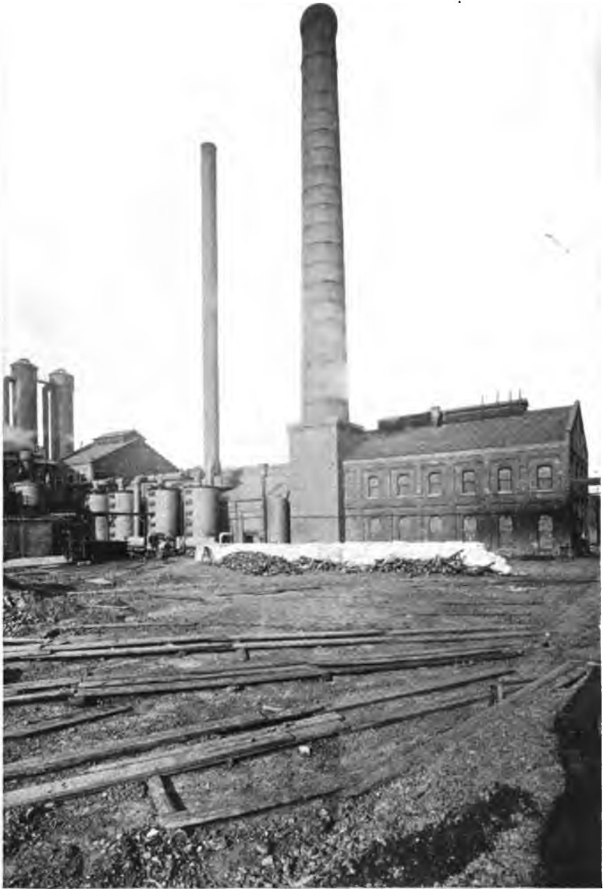
Peoples Gas, Light & Coke Co., Chicago, Ills., operating Heine Boilers.
