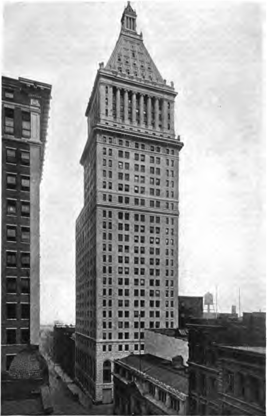
Union Central Life Insurance Building, Cincinnati, Ohio, equipped with Heine Standard Boilers.
