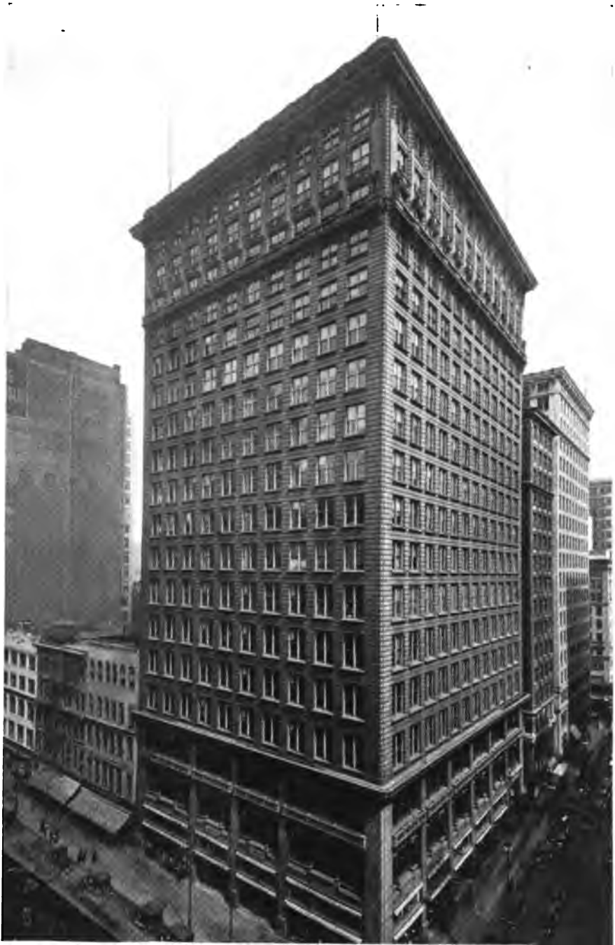
Lytton Building, Chicago, Ill., containing 1500 H. P. of Heine Standard Boilers.
