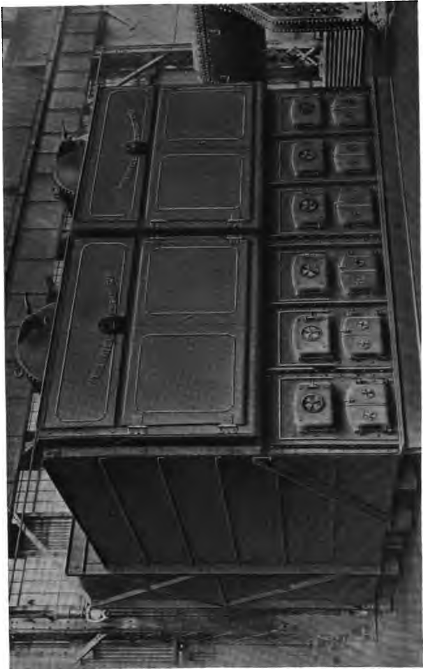
Two Heine Standard Boilers with Dredge Boat Setting.
