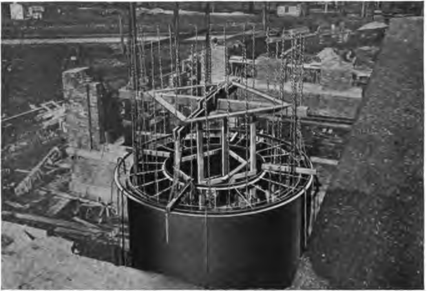
Fig. 110. Steel Forms and Reinforcing Rods in Place to Receive Concrete.
