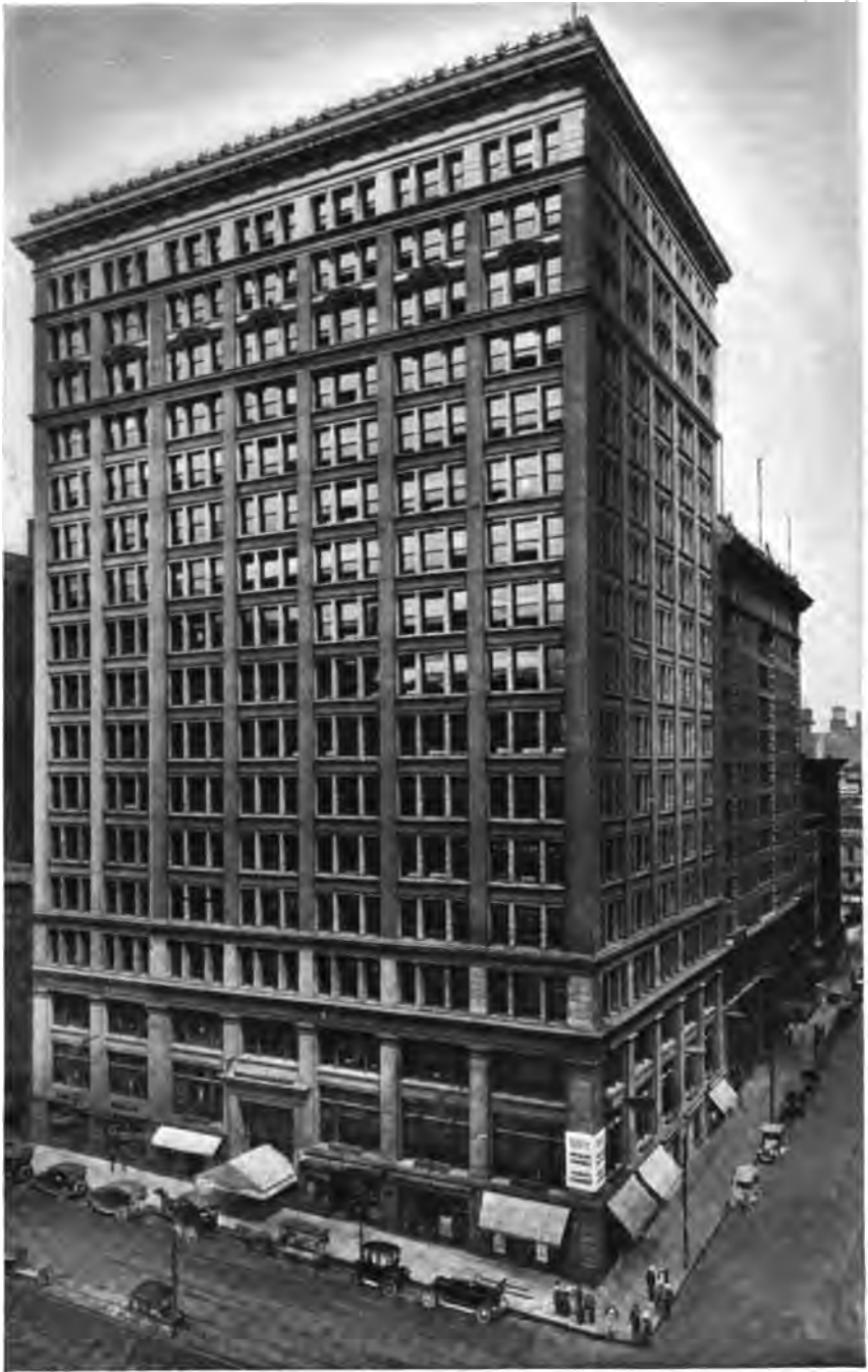
Union Trust Building, Cincinnati, Ohio, equipped with Heine Standard Boilers.
