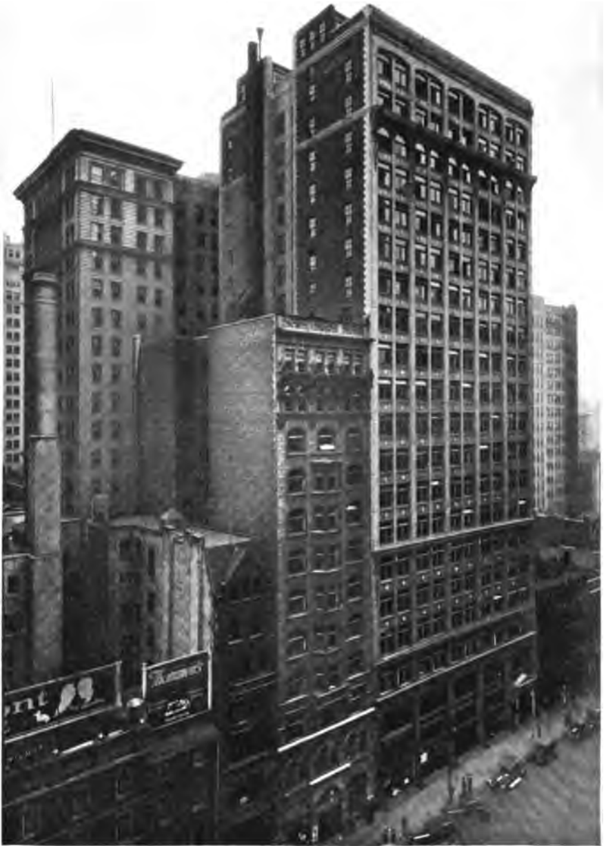
Finance Building, Philadelphia, Pa., equipped with Heine Boilers.
