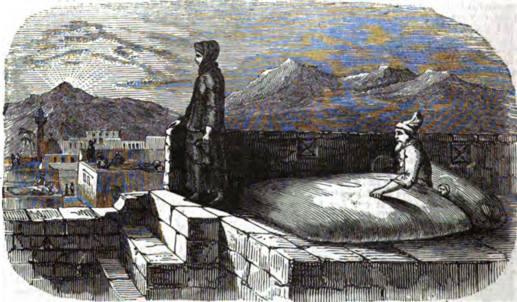
EASTERN DORMITORY ON THE HOUSE-TOP.
