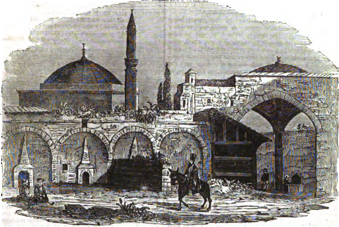
RUINED CARAVANSERAI AT HAFSA.
