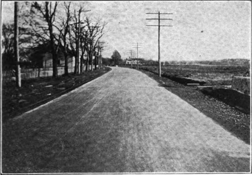
COMPLETED BITUMINOUS CONCRETE SURFACE — PUTNAM PIKE.
