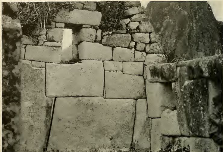
THE WALLS ARE BONDED BY A CLEVER USE OF INTERLOCKING ANGLES
