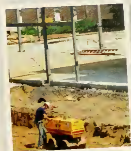
Construction at the Shoppes at La Salle
