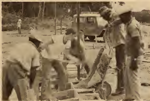
During January, fourteen Centenary students and Dean August Aamodt traveled to the British Honduras where they constructed a school in the wilderness for the native children of this jungle area. The people are poor and there would have been no school except for the help of the Centenary work-camp group.
