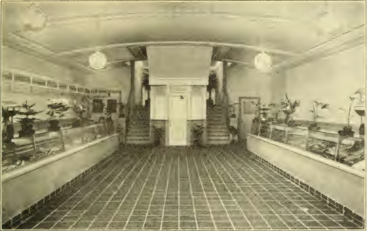
This illustration shows the basement of the new Wm. Davies Co. store, described in the preceding pages, where are situated the fish and grocery departments. Notice the spacious stairways leading from the ground floor.
