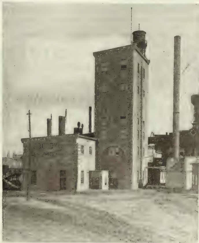
THE HOME OF THE E. B. EDDY CO.'S GIANT SULPHITE PULP DIGESTER
