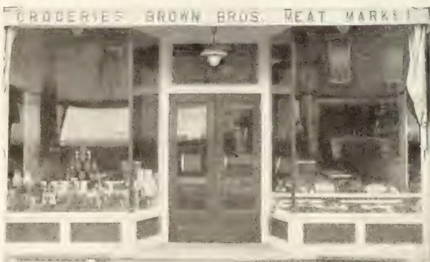
Exterior of Brown Bros. store, Owen Sound. Showing the cooling system installed in the window
