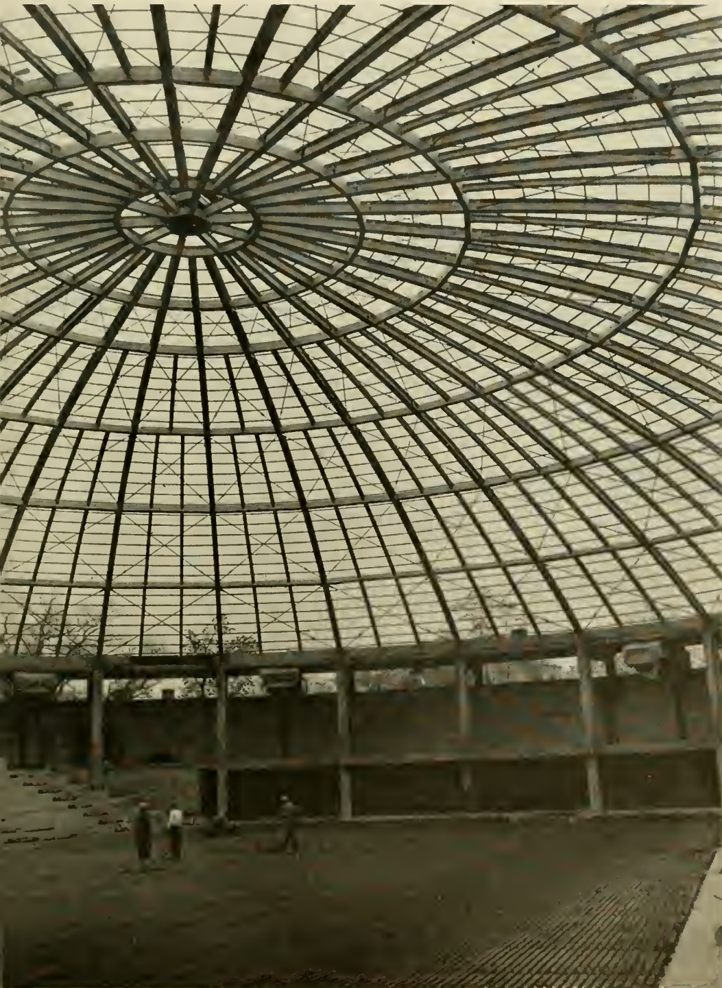
LAYING 10 MILES of brine pipe was only one of many spectacular construction operations.
