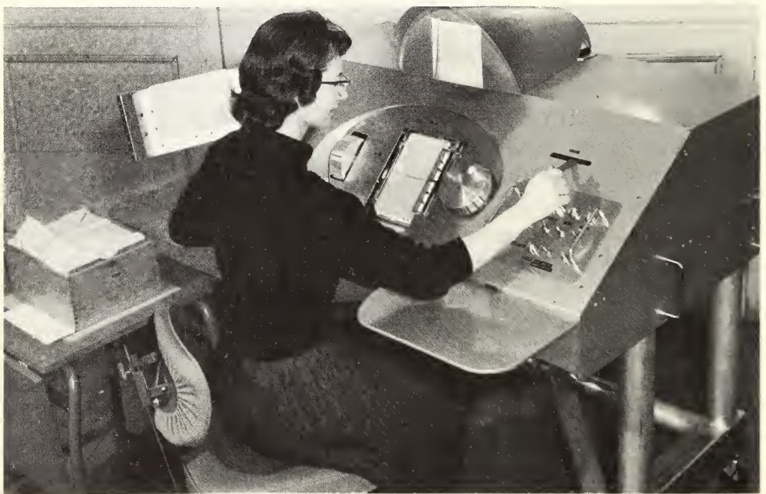
Microcite, a close-coupled searching machine developed for use with the NBS punched-card (peek-a-boo) instrumentation index. The operator can locate references, view abstracts on the screen at the top, and make copies of the selected abstract automatically (page 123).
