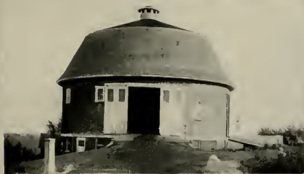
Dairy Demonstration Barn
