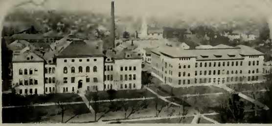
Bird's-eye View of Engineering Group
