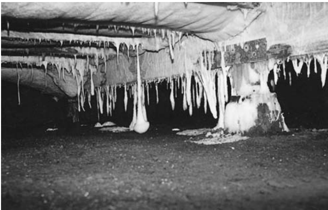
Fig. 14.6. Wood decay in recently constructed home by unidentified wet rot fungus. Photograph courtesy of Luis De La Cruz (De La Cruz Wood Preservation Services, Van Nuys, CA).
