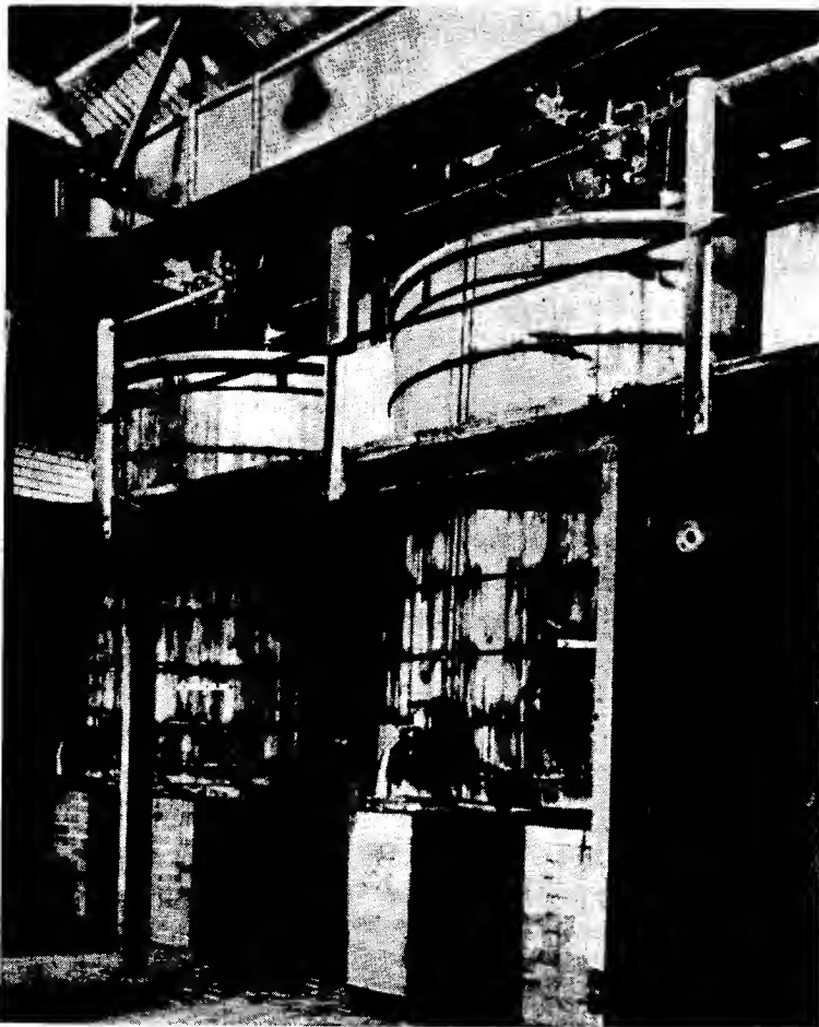
FIG. 26. Cyclonite boiling vats [55].
